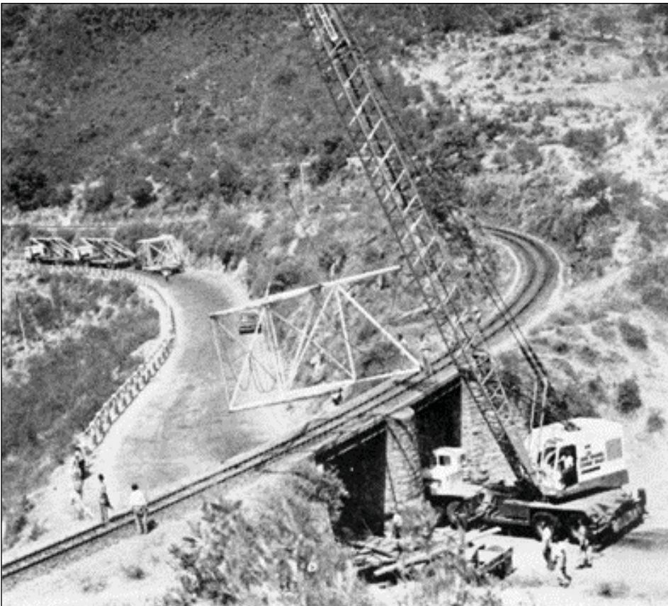
Support structures for the iconic STONEHOUSE antennas are lifted over a railroad bridge along the Asmara-Massawa road, 1964-1965. Public Affairs Office, United States Army Garrison, Kagnaw Station
