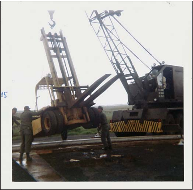
Site forklift sinks into the ground during installation of the 150' antenna. Handwritten captions read, "After this we should have quit," "We didn't," and "Motor pool to the rescue." Courtesy of William Semenuk
